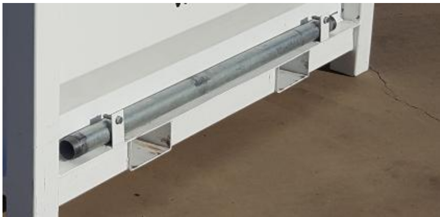
Figure 19: Vent pipes secured to tank
