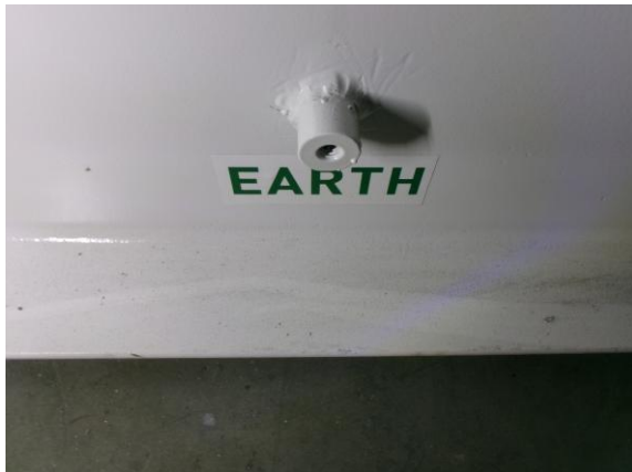
Figure 30: Earthing connection
