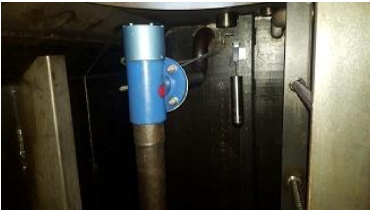
Figure 14: Hydraulic overfill protection valve
