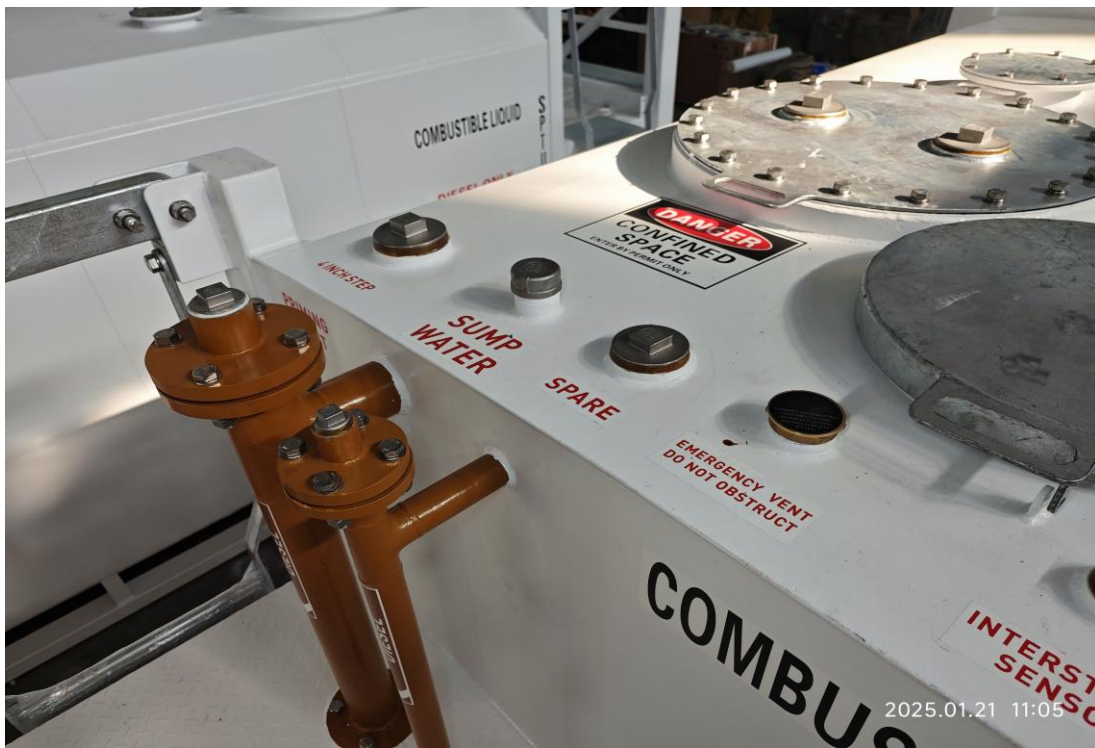
Figure 7: 1.5" & 3" Priming Point (Brown pipework)
