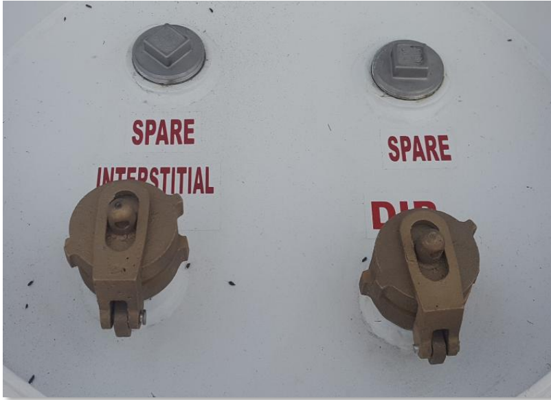
Figure 29: Dip point inside hatch
